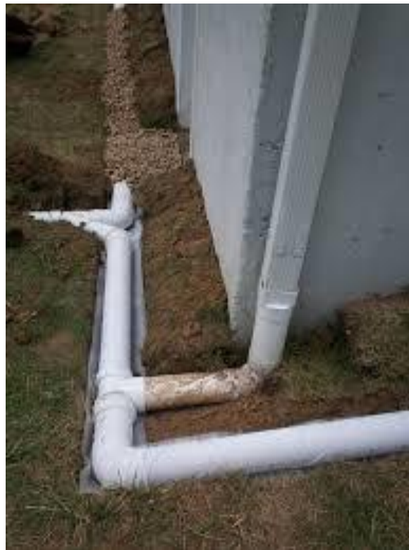
Example of an underground drainage pipe installation made of PVC designed to be connected to the gutters
